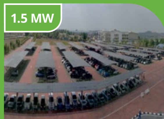
3. Covered carpark and motorcycle area
