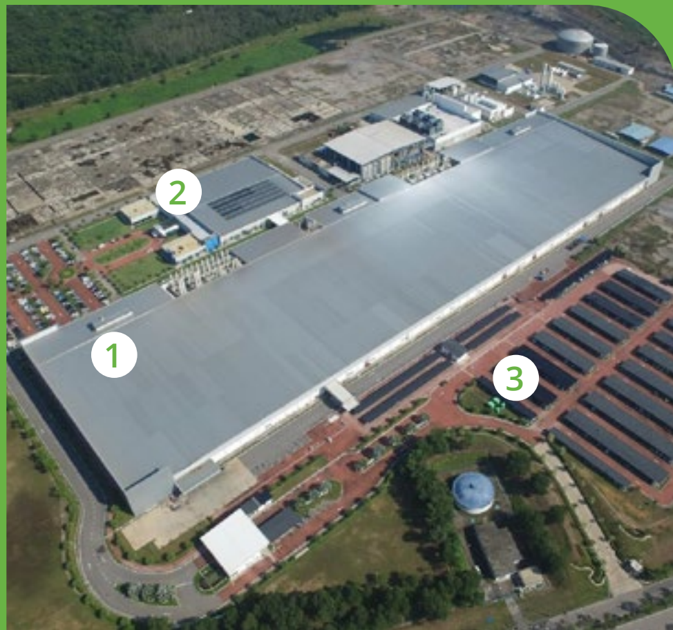
1. Future planned – FAB rooftop
